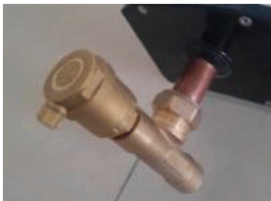
Exhaust valve connection
